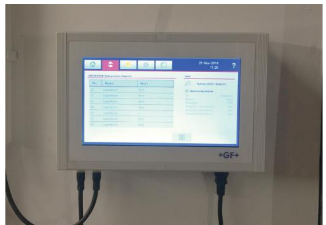
The integrated sanitary technology is easy to operate from the Hycleen Automation Master control unit. The panel is connected to controllers, which precisely control the individual valves and sensors.
