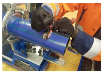
Use a tool to cut the protection layer. To make the removal easier it is better to remove maximum 50mm wide longitudinal slices at a time.
