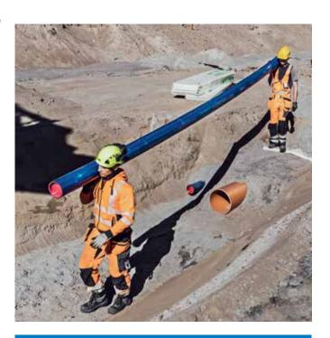
NOTE! The protection layer protects the barrier layer, it does not protect the PE pressure pipe against mechanical stress. A damaged protection layer is a risk for water contamination.
