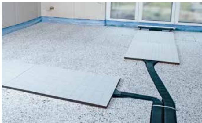
Uponor Comfort Air is installed together with the Pluggit Pluggflex ventilation ducts. The corresponding adapters enable professional integration into the ventilation system.
