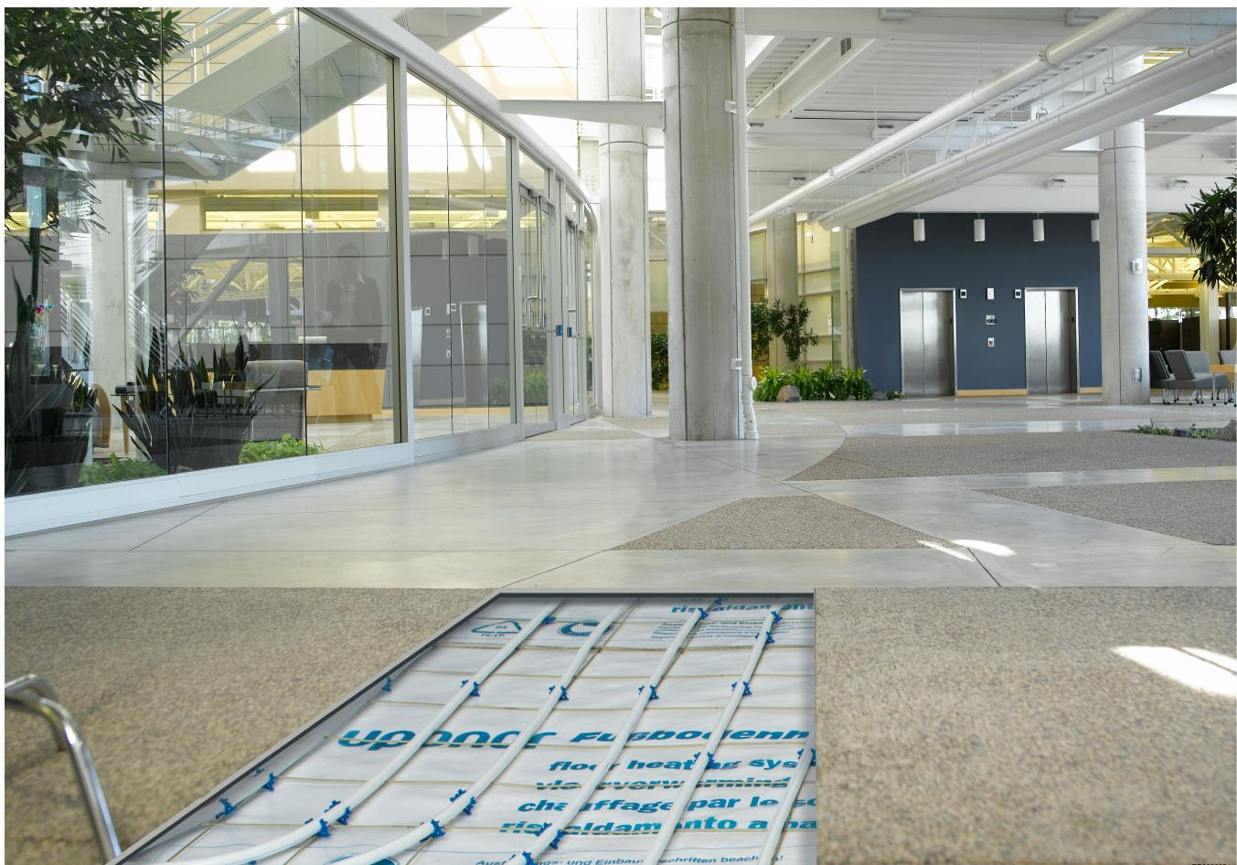
The Uponor Classic is a wet installation underfloor heating and cooling system for different floor structures in residential and commercial buildings. The Uponor Classic has three different mat grids that allow the spacing between heating pipes to be adjusted according to heating requirements. The coated supporting elements and robust pipe holders reliably secure the piping system and ensure the screed surround is optimal at the heating level.
