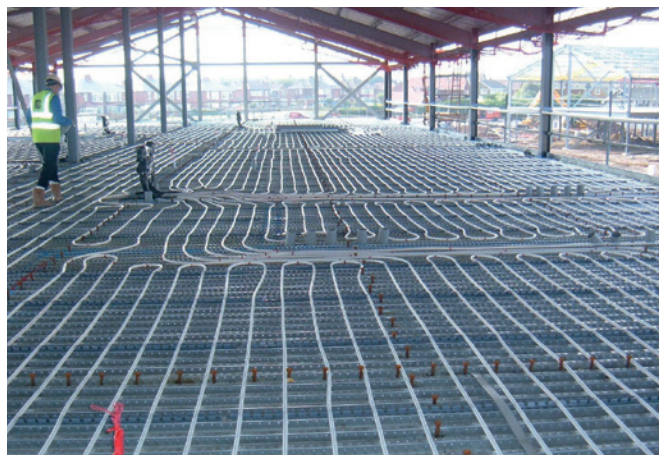
Uponor Contec in Trapezblechdecke.
