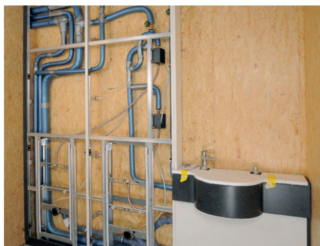
The compact design of Sanipex MT enabled complete prefabrication, which saved time and thus ensured that the deadline was met. [Picture credits "Hug GmbH und Co KG"]
