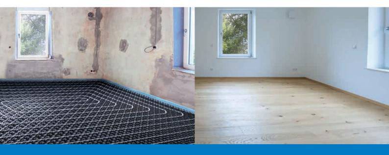
>>> Heat pumps are becoming increasingly popular and radiant heating systems are the ideal cost-effective, energy-efficient solution for heating our homes, because heat pumps work best at low supply temperatures and are most efficient when they provide heat over a large area.
