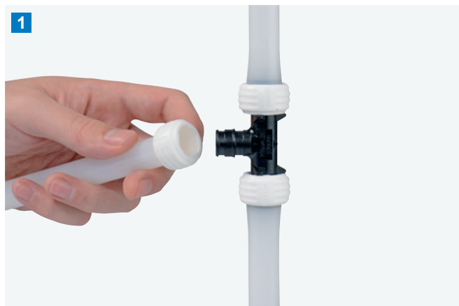
Add the Q&E ring on to the end of the pipe
