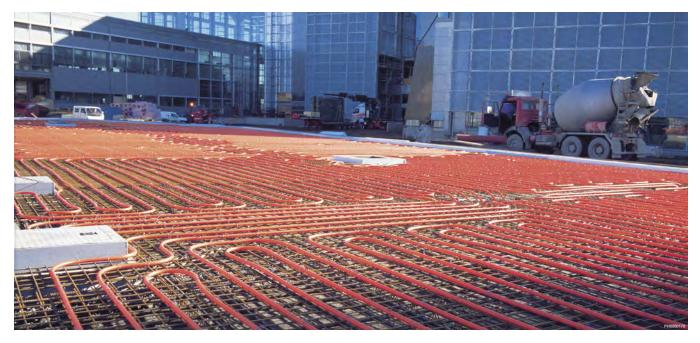
The Uponor Meltaway system is normally installed just underneath the surface layers of the structure. The structural requirements and load-bearing characteristics of such areas must be determined to ensure that predicted loads will not cause the piping to break. The Uponor Meltaway system will not reduce structural requirements.
